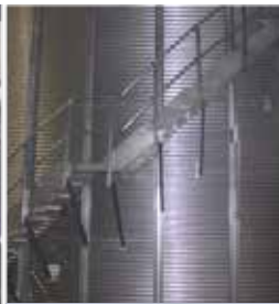
4 SPIRAL STAIRWAY Distributed spirally around the silo.
