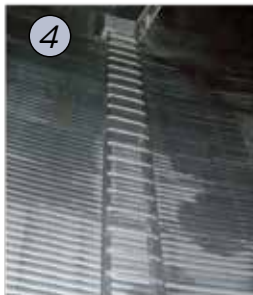
6 INSIDE LADDER a) It connects access door on the slope to the ground. b) As an option, it may connect the inspection door to the ground.
