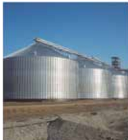
FLAT BOTTOM SILOS (OR WITH CONICAL CONCRETE FOUNDATION) FOR LONG TERM STORAGE OF LARGE QUANTITIES OF GRAIN, SEEDS...
