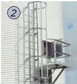
2 LADDER TO ACCESS DOOR Includes a support platform.
