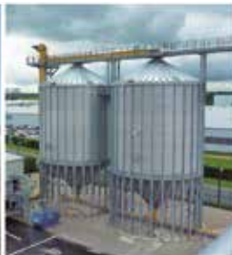
SILOS WITH LOWER STEEL HOPPER, WITH 45° OR 60° DEGREES DEPENDING ON THE FLOWING OF THE PRODUCT STORED. DISCHARGE BY GRAVITY
